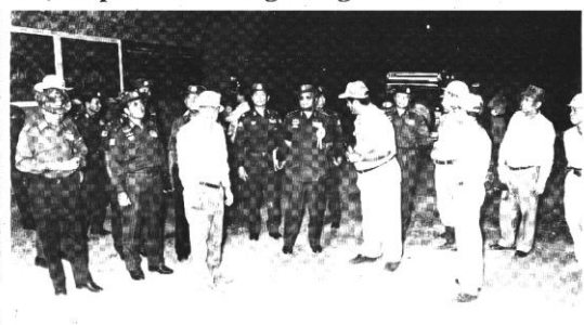
Senior General Than Shwe inspects preparation to lay concrete on upper interior surface of the diversion tunnel at Mone Creek Multi-purpose Dam.—MNA
